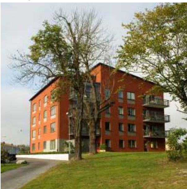
Apartment Building, Hallstahammar (source: NCC)
